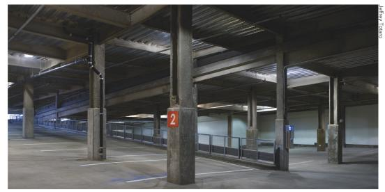
All the steel columns in the enclosed and mechanically ventilated garage were encased in concrete for impact protection.
