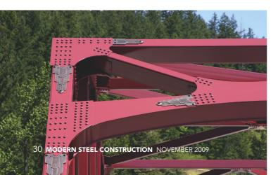
Art elements, such as the decorative bronze plates attached to the bridge structure, combine with the bolt connections to make the Mount Si Bridge a distinctive and aesthetically pleasing structure.
