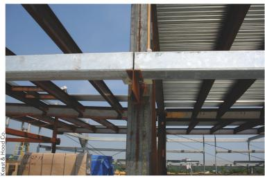
To accommodate the variety of building skin systems on this project, numerous details were developed, such as this galvanized tube for the front façade.
