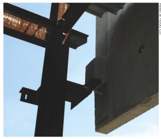
With the seats for the wall panels already in place on the columns the panels could be put in place much earlier in the process.
