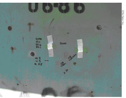
This coating damage is the result of destructive adhesion tests on the east exterior fascia girder of the Windgap Bridge, near the north abutment. All indicate excellent adhesion.
