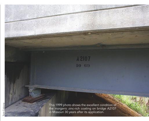
Evaluation Program (NTPEP). Suppliers of coatings to the bridge painting industry are now required to have their products tested in accordance with the AASHTO NTPEP testing standard for Structural Steel Coatings (SSC). In these laboratory "torture tests," the performance of candidate bridge coating systems is evaluated using tests identical to those required to qualify the IOZ/E/U system described above.
